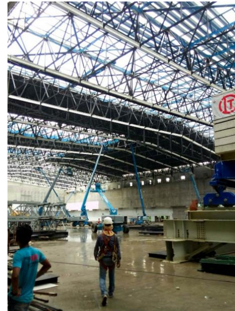
Genie was the only brand to meet the low Occupied Floor Pressure requirements
